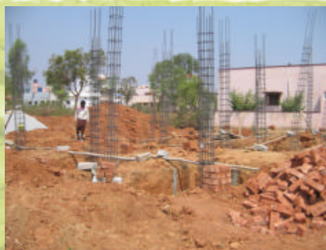
The structure as on first week March 2010
