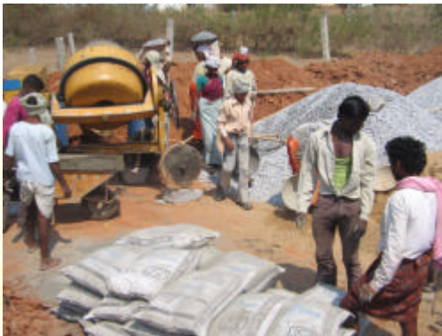
Work in Progress at Construction site
