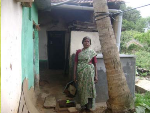
Notice the square pit below the green tap at the bottom of the RWH tank. The pot or water tube could be used to draw water.
