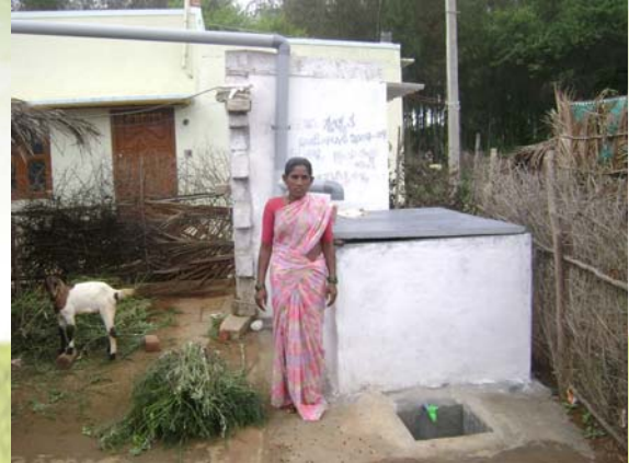
One of the 61 Rain Water Harvesting systems sponsored by the guests at Arjunabittahalli Village
